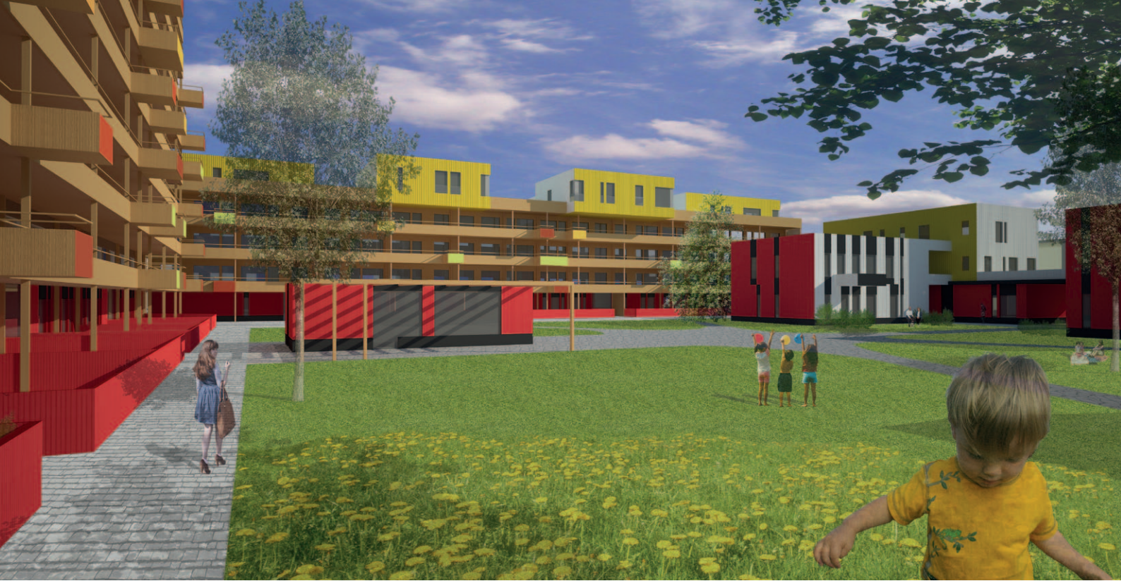
The new balcony belt will give the apartments considerably more usable space. The balconies can be glassed in entirely or partly, which will increase their use.
