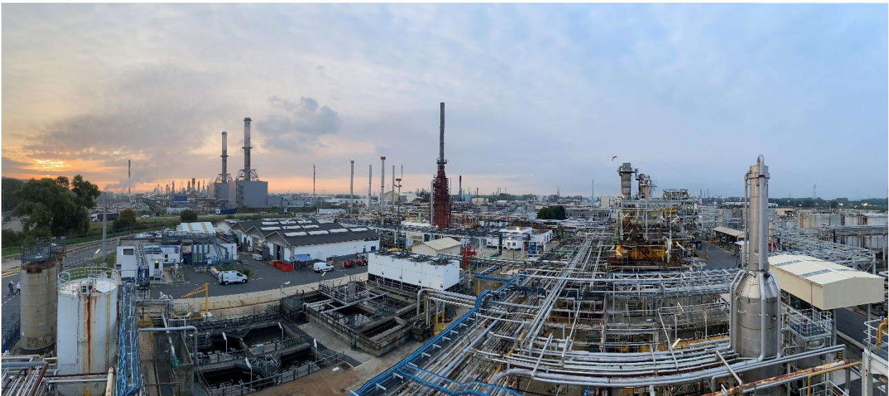
Figure 1. A general view of the Chevron Oronite plant.
